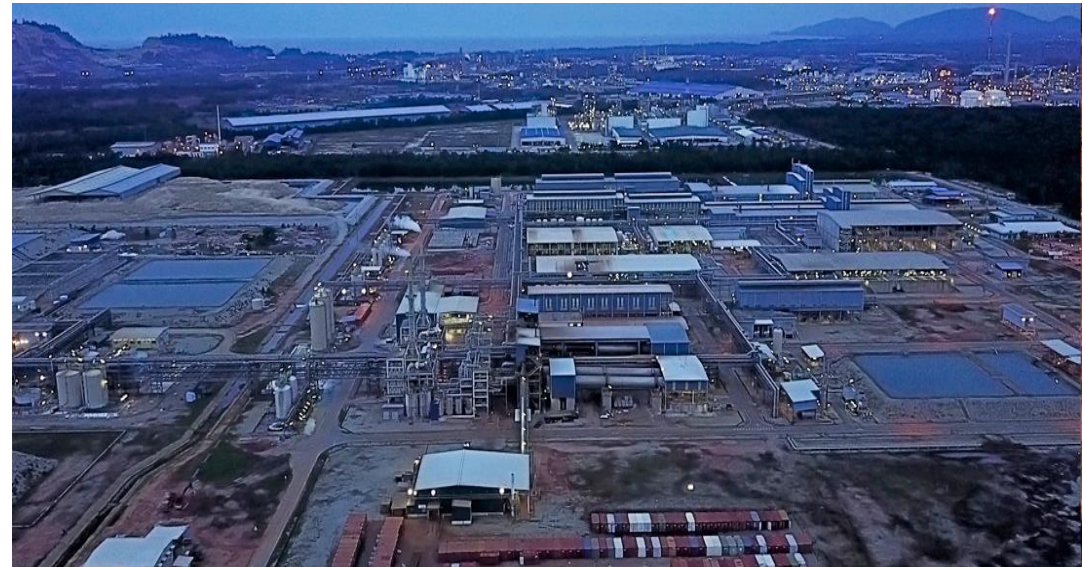
Lynas Corporation 's cracking and separation facility Kuatan , Malaysia
